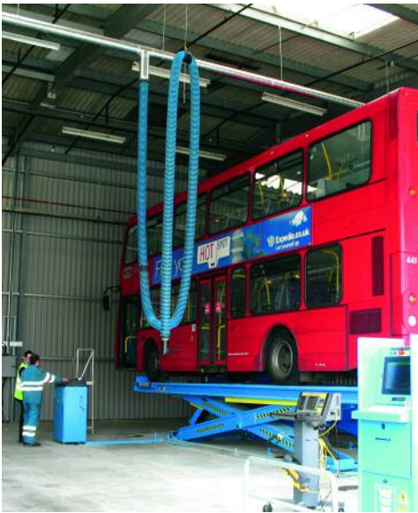
The scissor lift at the new depot: £5.5million was invested refitting the building including rainwater harvesting from the roof for the bus wash.
